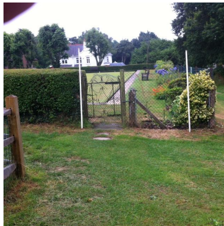
SE corner showing position of widened gate
